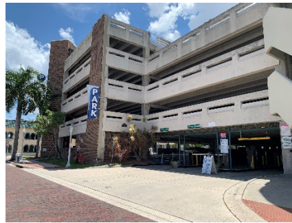
Main Street Garage: 2286 Main Street
